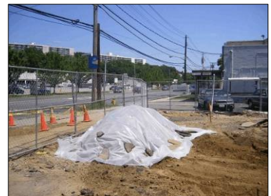
Contaminated Soil Removal
